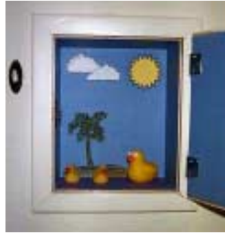
Figure 3: Current condition of an embedded milkbox in a building from 1940
