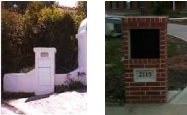
Figure 6:dValut boxes covered with stucco and brick
