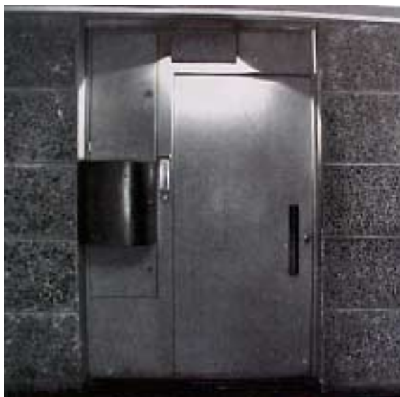
Figures 5 and 23. Delivery Area in L'unité d'Habitation. Exterior picture and plan view
