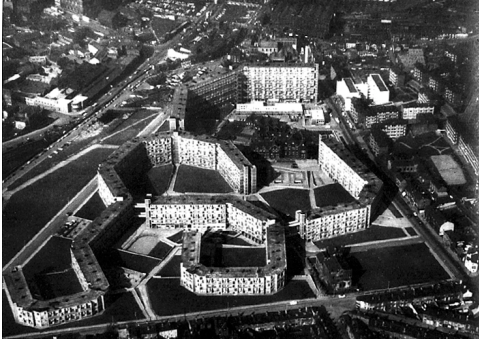
Figure 24: Aerial view of Park Hill Source: All Pictures from the Book Park Hill, what's next? By Andrew Saint, Published by the Architectural Association in 1996
